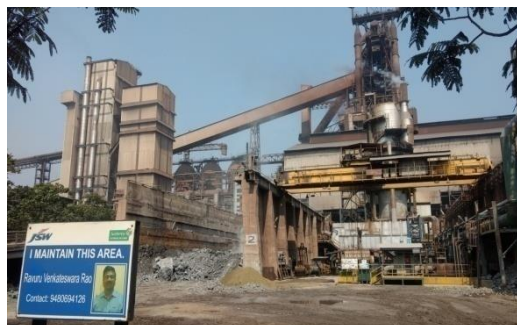
Fig.2 Blast furnace plant
