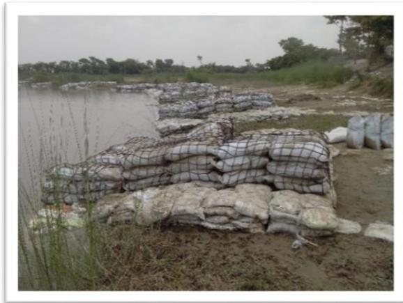
Figure 2: Polymer Rope Gabion
