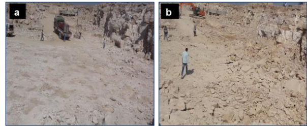
Figure 5 Field Photo of the Study area (a) before blast and (b) after blast.
