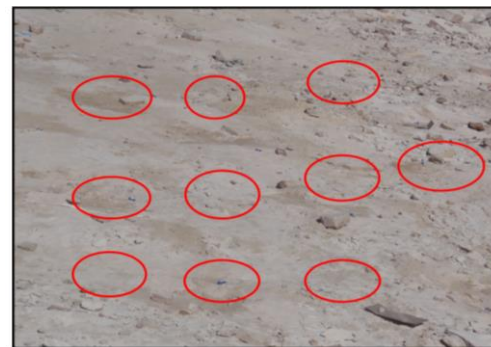
Figure 3 Filed Photo of Blast holes.
