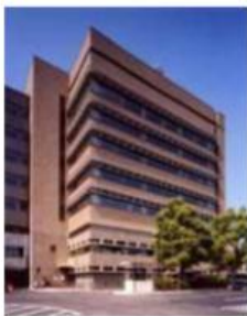
Photo 4 Building external view
