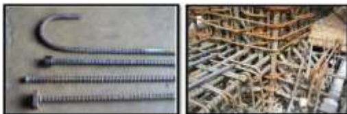
Fig.1.1(a): Various headed bars Fig.1.1 (b): Congestion of Beam-column joint
