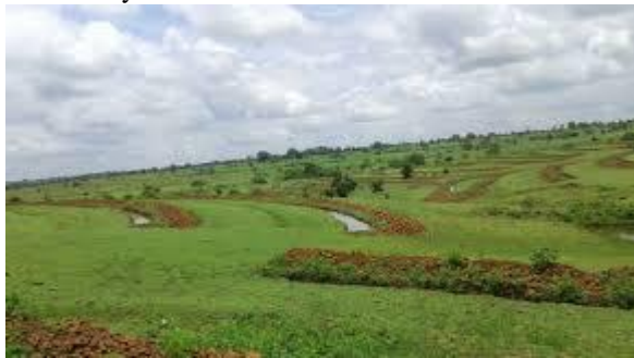
Continue counter trenches
