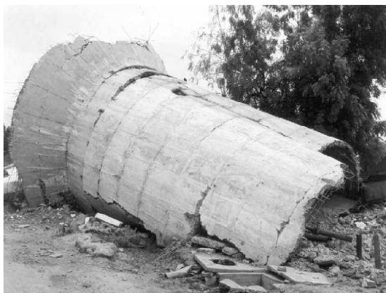
Figure: 1.4. Collapse of water tank in Bhuj
