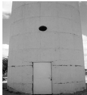
Figure: 1. 3. 200 kL Bhachau water tank which developed circumferential cracks up to one-third height of the staging. Severe cracking at the junctions of the first two 'lifts'.
