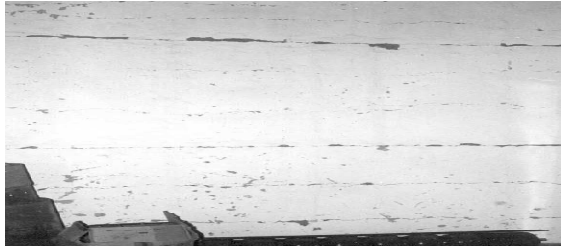
Figure: 1.1. Cracks are 'through' the shell thickness as seen from inside the shaft of 1000 kL Anjar Nagar Palika Tank
