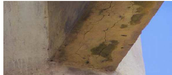
Figure: 1.6. Crack in soffit concrete under Side the staging beam of tank
