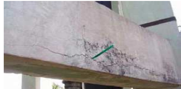
Figure: 1.7.Crack in soffit concrete along the entire length of a staging
