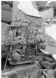
Figure: 1.2. Poor detailing of column-brace joints for Manfera tank
