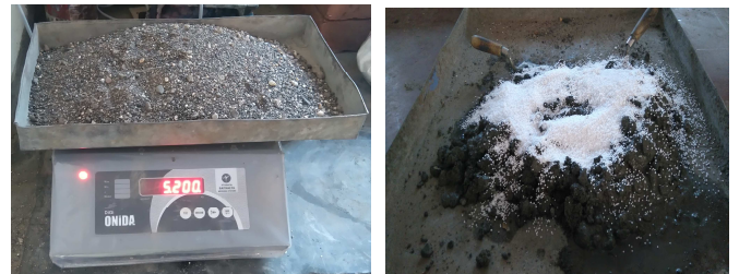
Fig 1- Showing Weight Batching and Mixing of concrete Materials.
