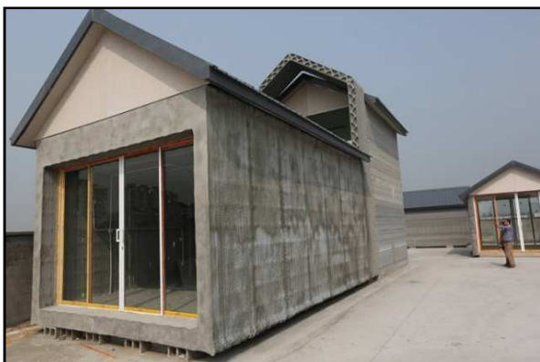
Fig. 8 A typical house constructed using 3D printing technology by WinSun Corporation, China
