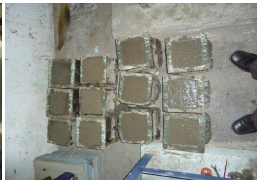
Casting Of Concrete Cubes
